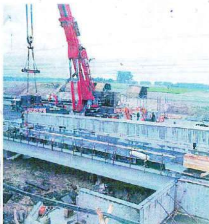
The complexity of the PX 112 job site
