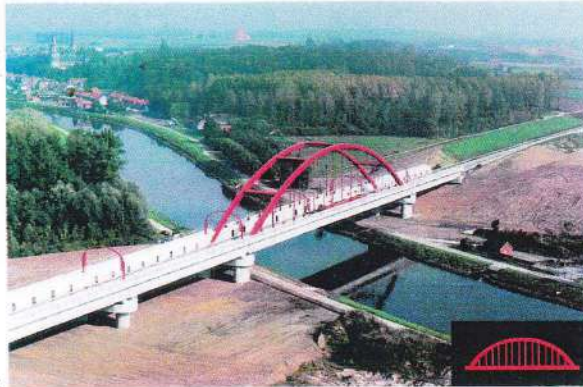
Viaduct over the Escaut river in Antoing
