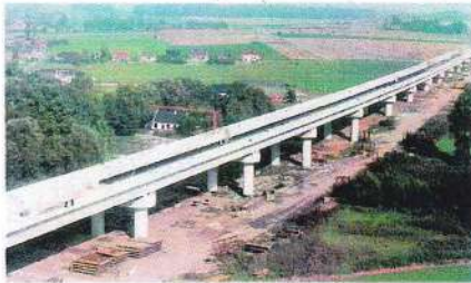
The Arbre viaduct being waterproofed
