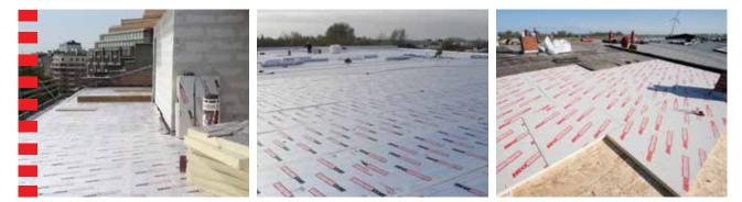
IKO enertherm is used for the thermal insulation of flat roofs.
