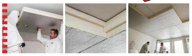
IKO enertherm is used for the insulation of underground spaces and basements.
