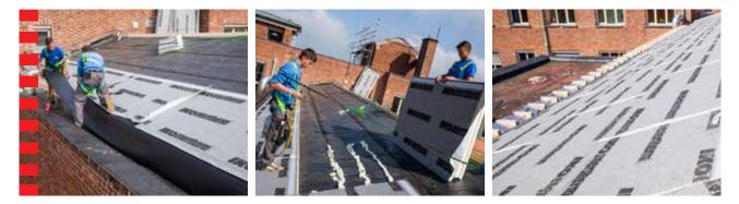
IKO enertherm is used for the thermal insulation of pitched roofs on the rafters or on the trusses.
