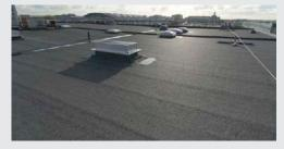
**DERBIBRITE® NT**, with a highly reflective coating, acting as a "passive cooler", thus allowing cost savings on cooling energy costs
