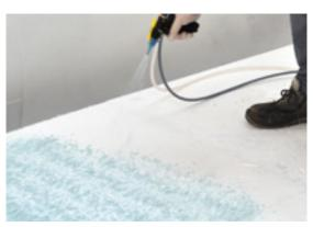
Pict. 2: The adhesive  $\mbox{RENOLIT}$  DUALFIX\_{\mbox{BIOBS}} is atomized by means of a spray gun.
